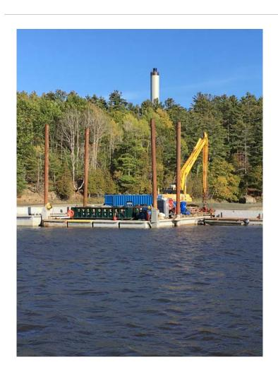
Removal: Excavation or dredging of contaminated materials to remove contamination.
